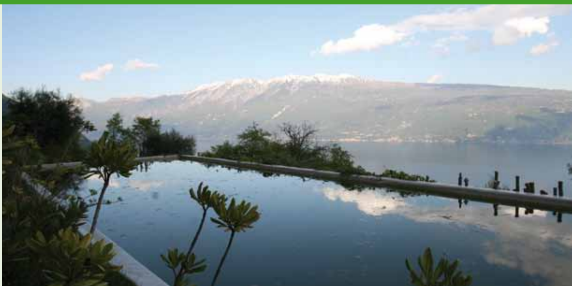
View of the Lefay Resort & SPA Lago di Garda rainwater collection tank
