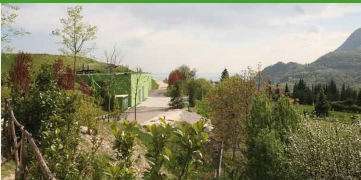
View of the Lefay Resort & SPA Lago di Garda Energy Plant
